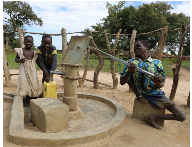
People living with disabilities can easily use the borehole because it has a seat for use while pumping and a platform for resting a water container before putting it on a wheelchair. Photo: WaterAid/James Kiyimba
